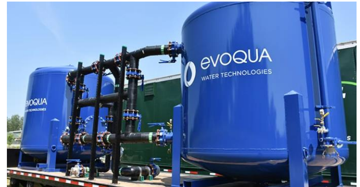
Mobile water treatment system
